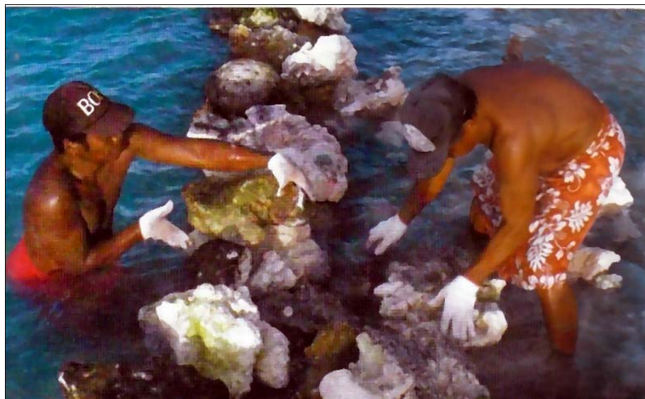
Building a new sea wall to protect a village
