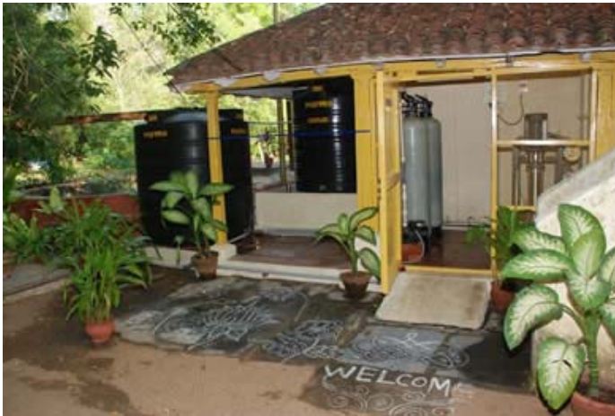
The reverse osmosis plant ensuring pure water for the residents and visitors at Adyar.
